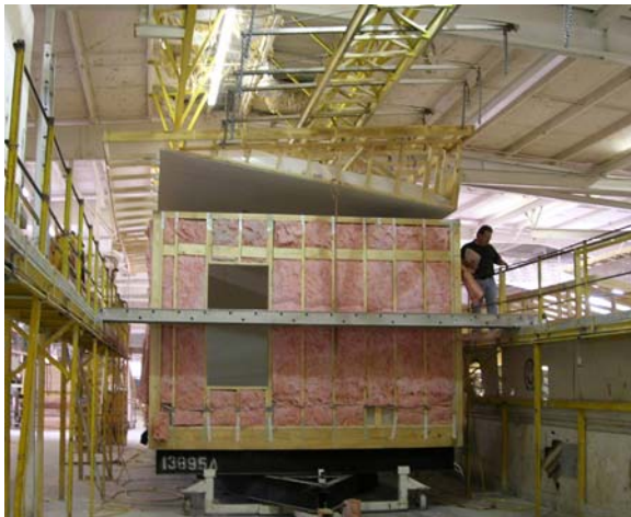
Pre-fab module in production line
