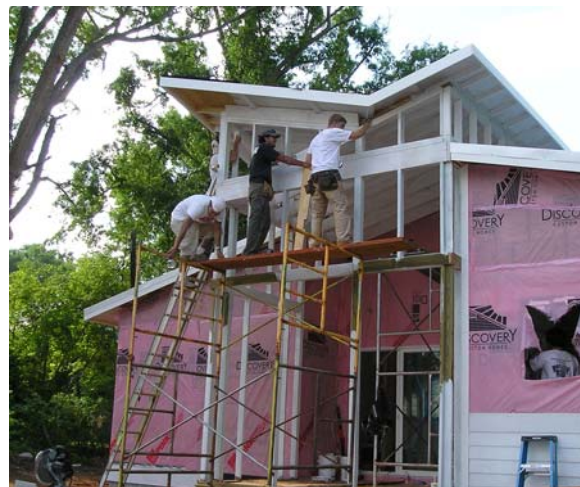
Center bay under construction
