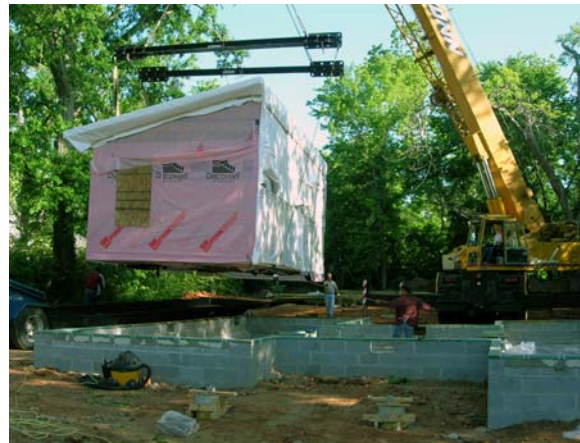
Setting modules on the foundation
