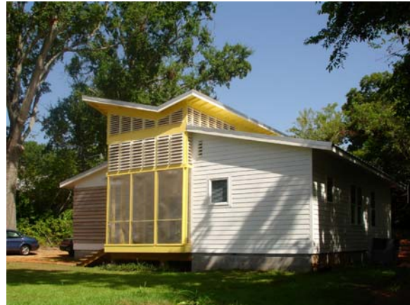
Front view of completed home
