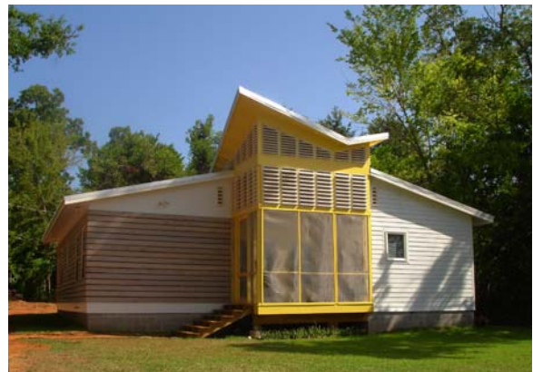
Front view of completed home
